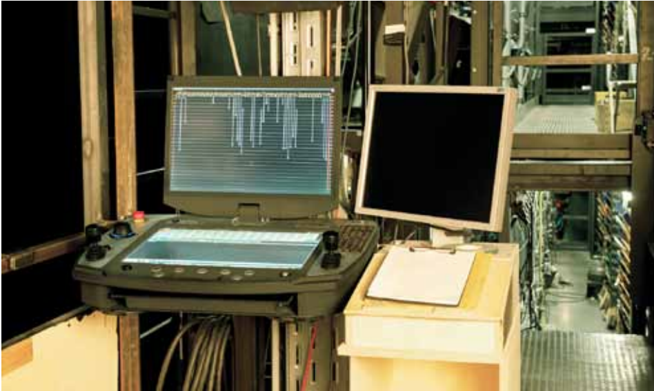
Figure 2: After a modernization, stage technology at Theater Duisburg is now mainly operated by means of fixed OpenCue consoles with two 22-inch touchscreens
