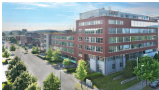
Figure 1: Vector has invested in bricks; the next buildings are already planned
